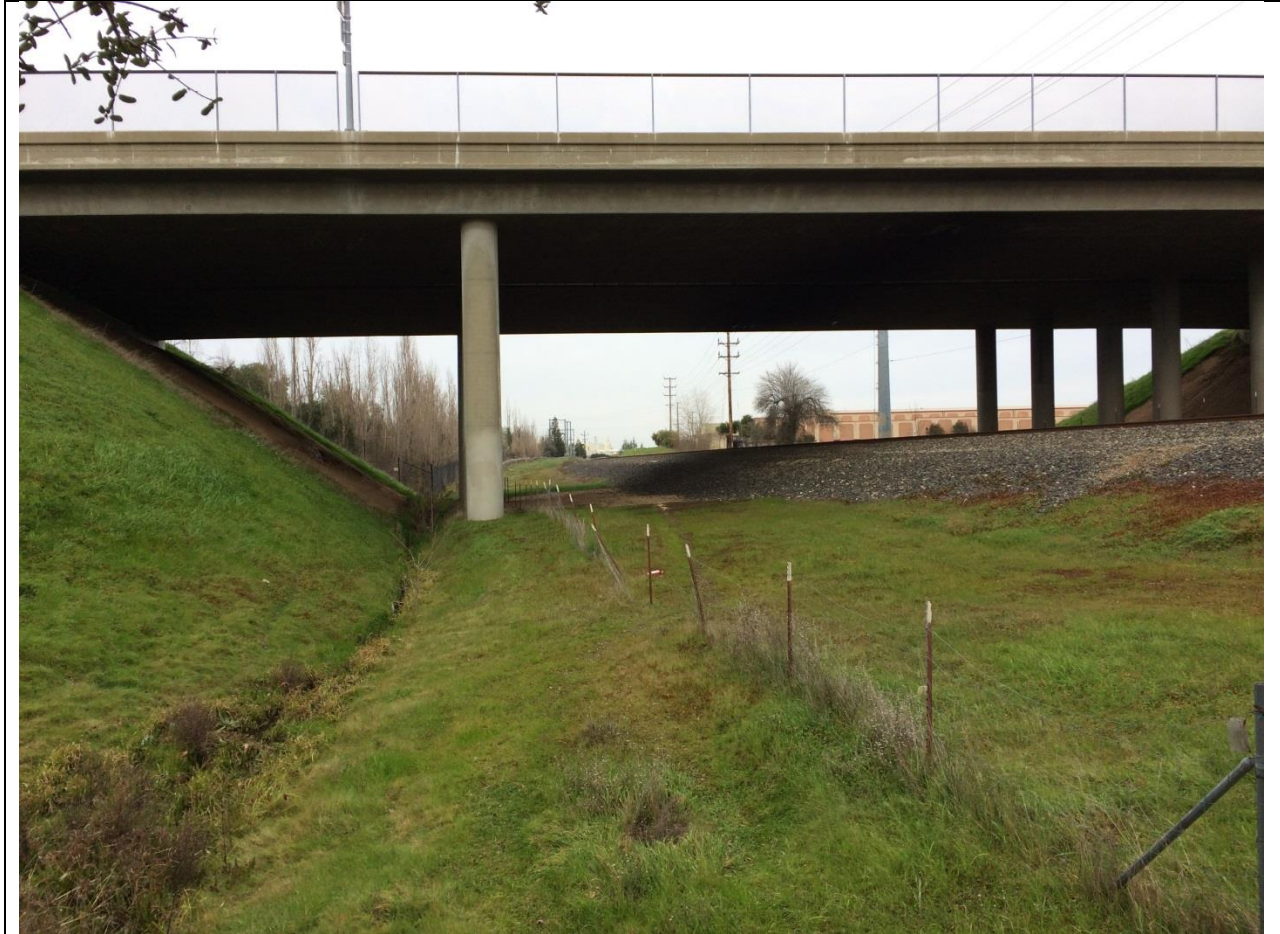
Photo 13. Looking northwest adjacent to the existing UPRR right-of-way (right side of fence), west of Washington Boulevard, north of the Andora bridge, and south of Pleasant Grove Boulevard (overpass structure). Photo depicts ditch (on left) near north end of City open space preserve. Photo taken February 1, 2017.
