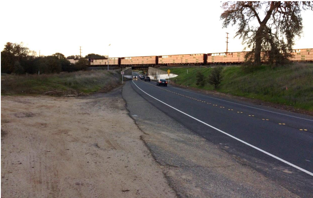
Photo 2. Looking north from the west side of Washington Boulevard, south of the Andora bridge, at disturbed/graded area (left foreground). Photo depicts narrow vehicle underpass (background) and proposed temporary access road (graded area, foreground) to proposed staging area. Sign to left of roadway indicates that pedestrian access is prohibited under the bridge. Photo taken December 6, 2016.
